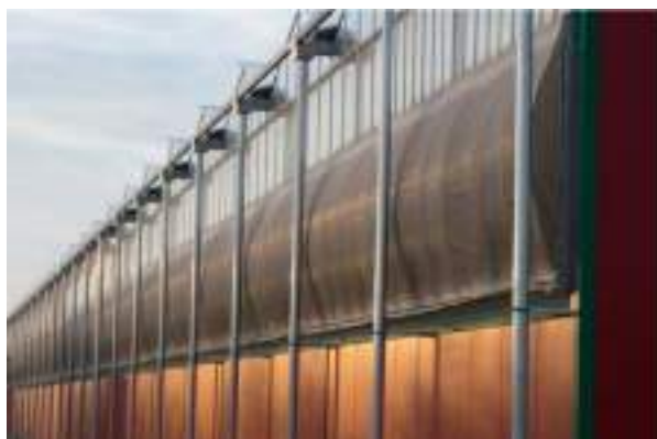
Fig. The SuprimAir greenhouse made by Certhon. Left: the roundish shape is a long window to let air into the corridor. Below that is a wet pad. Heating is also included.
