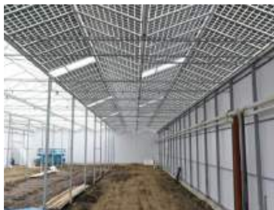
Hortisolar in Zevenbergen (NLD), 390 kWp.
