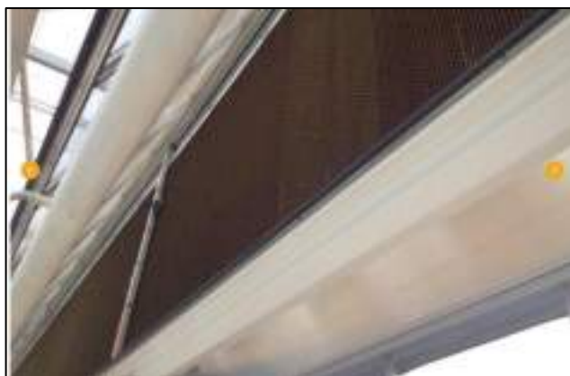
Fig. Interior of the air treatment corridor of an Ultra-Clima greenhouse from KUBO (NLD). Outside air can enter from the top and mixed with greenhouse air. The conditioned air is sucked into the grey boxes and then pushed into a sleeve. This is at D’Vine Ripe in South Australia.
