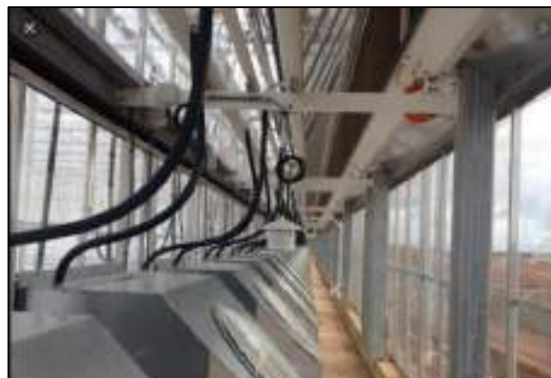
Fig. Interior of the air treatment corridor of an Ultra-Clima greenhouse from KUBO (NLD). Outside air can enter from the top and mixed with greenhouse air. The conditioned air is sucked into the grey boxes and then pushed into a sleeve. This is at D’Vine Ripe in South Australia.
