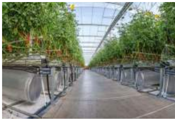
Fig. The SuprimAir greenhouse made by Certhon. Left: the roundish shape is a long window to let air into the corridor. Below that is a wet pad. Heating is also included.
