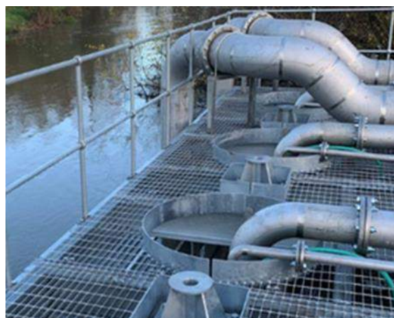
Fig. .... Heat pump extracts heat from a lukewarm source, e.g. greenhouse air (26 °C), or water in canal (16 °C) and transfers it to warmer water (e.g. 30 °C).
